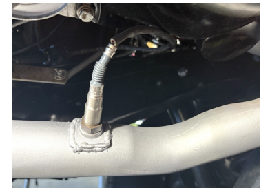
Oxygen Sensor Installed
