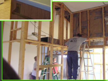
Tearing out walls and ceiling.
